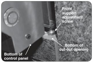
Fig. 21-1 Front support adjustment screws
