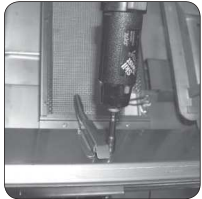
Fig. 4-2 Install new lighting tube
